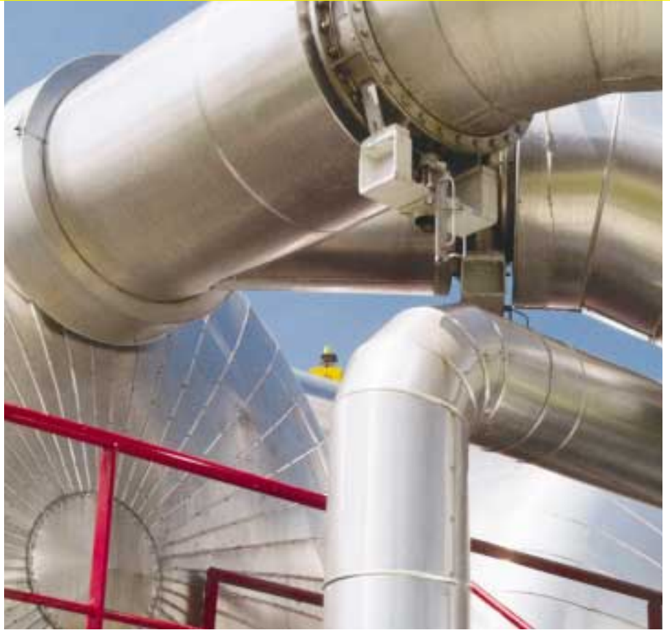
Actuator with hydraulic speed control
